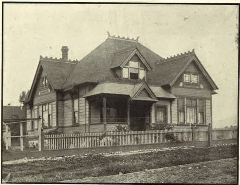
RESIDENCE OF WM. SHIPSEY, Corner Mill and Essex Streets.
